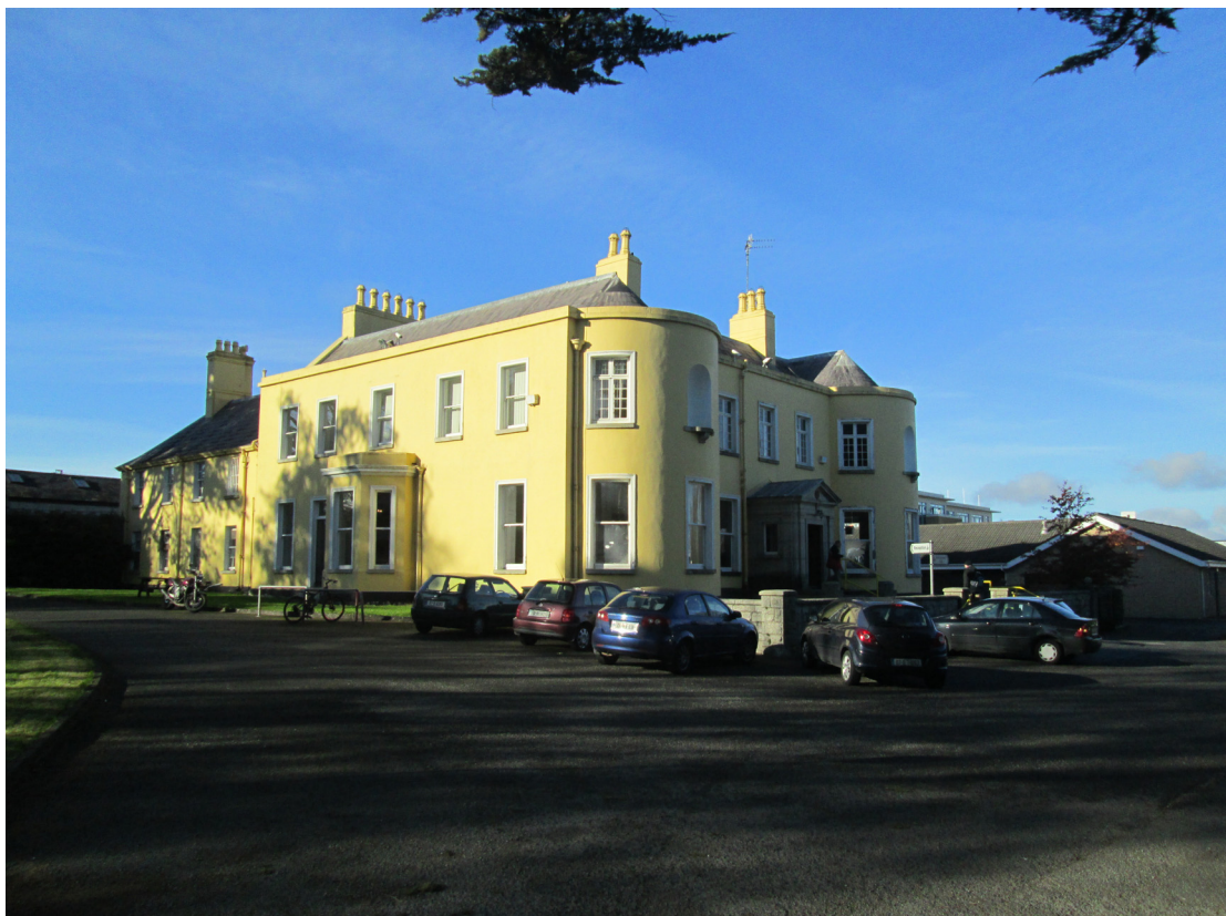
Figure 11.1 Burton Hall, Arena Road, Sandyford
